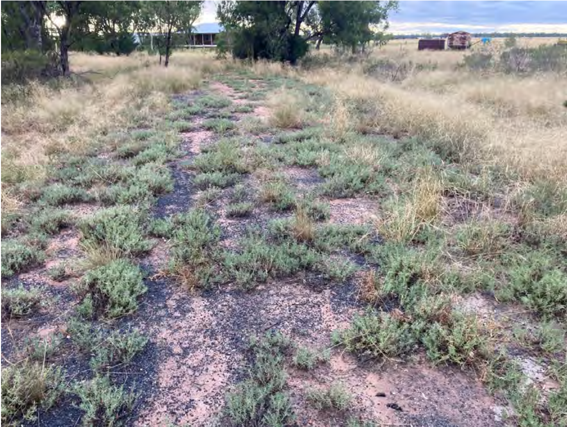
Photo 1: Existing track off the Newell Highway to the entry of site. D. Wall 2021
